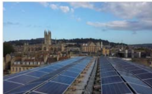
1 Lewis House Roof - Courtesy of BWCE
